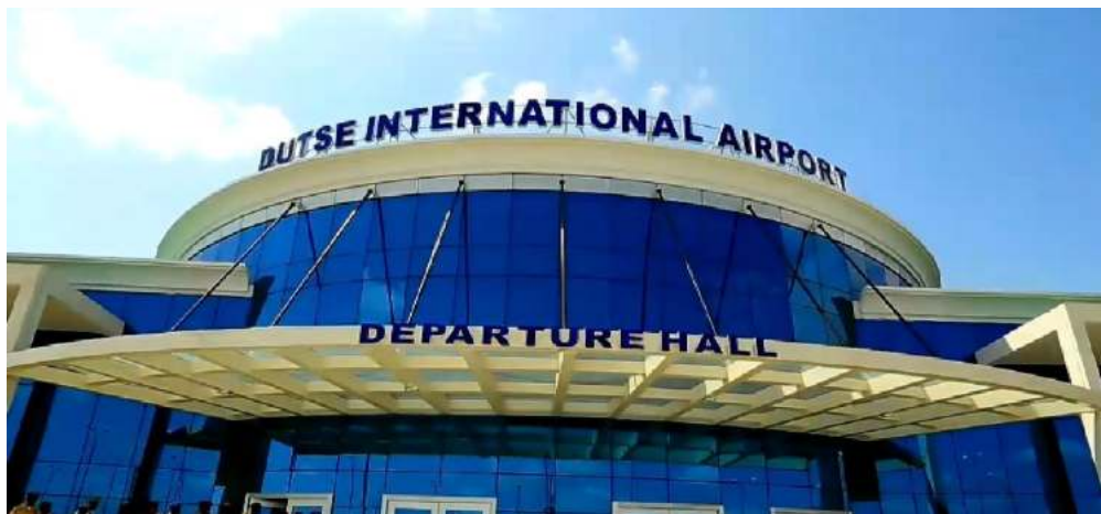
Dutse International Airport
